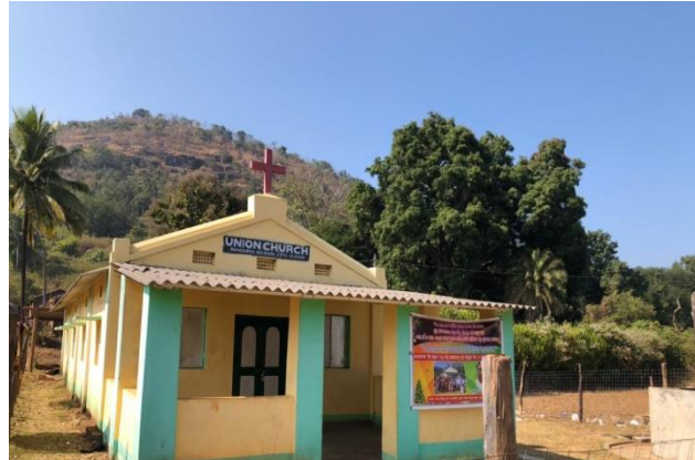
Figure 4:8 Prayer hall restored but services are yet to start normal.
